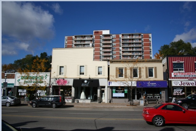
Figure B71 -Mainstreet building frontages
