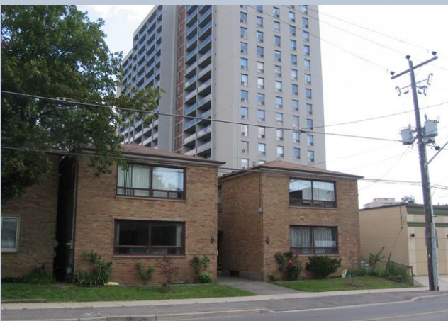
Figure B18 - Image of the Riverside Precinct
