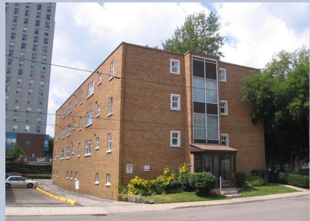
Figure B19 -Image of the Riverside Precinct
