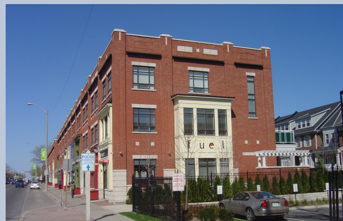
Figure B27 -Image of the existing mainstreet building
