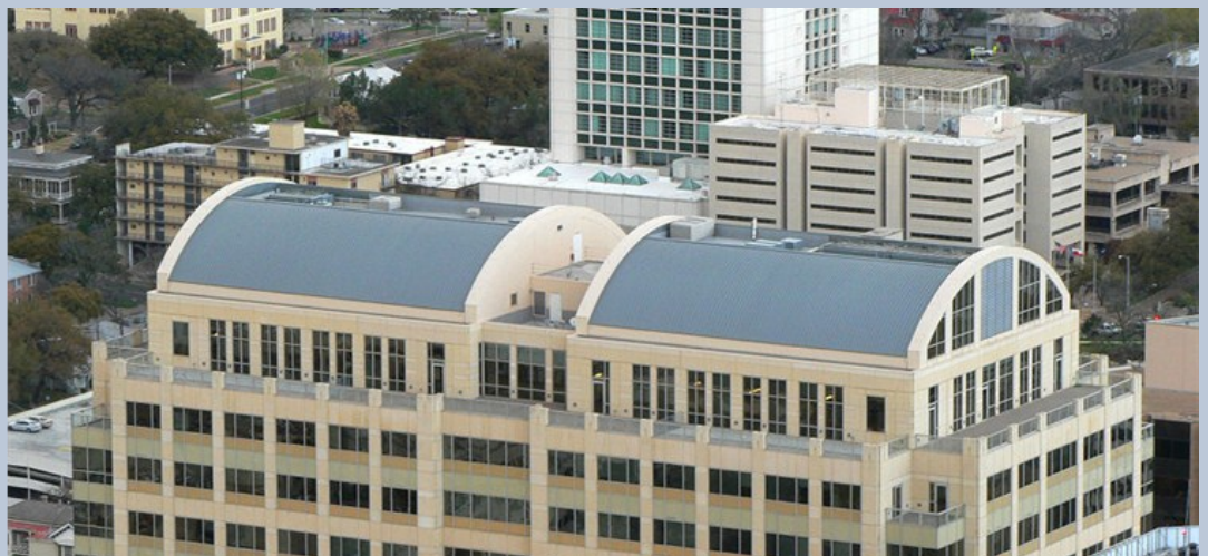
Figure B100 - Example of roof top mechanical that has been integrated and designed into the building
