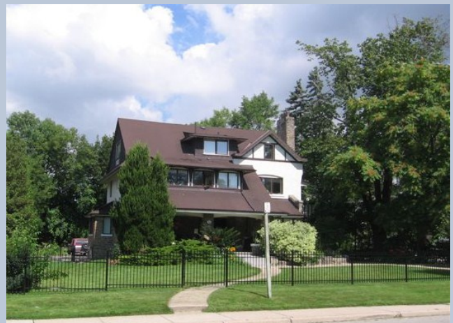
Figure B143- 84 High Street East, CG Hamilton House, Designated
