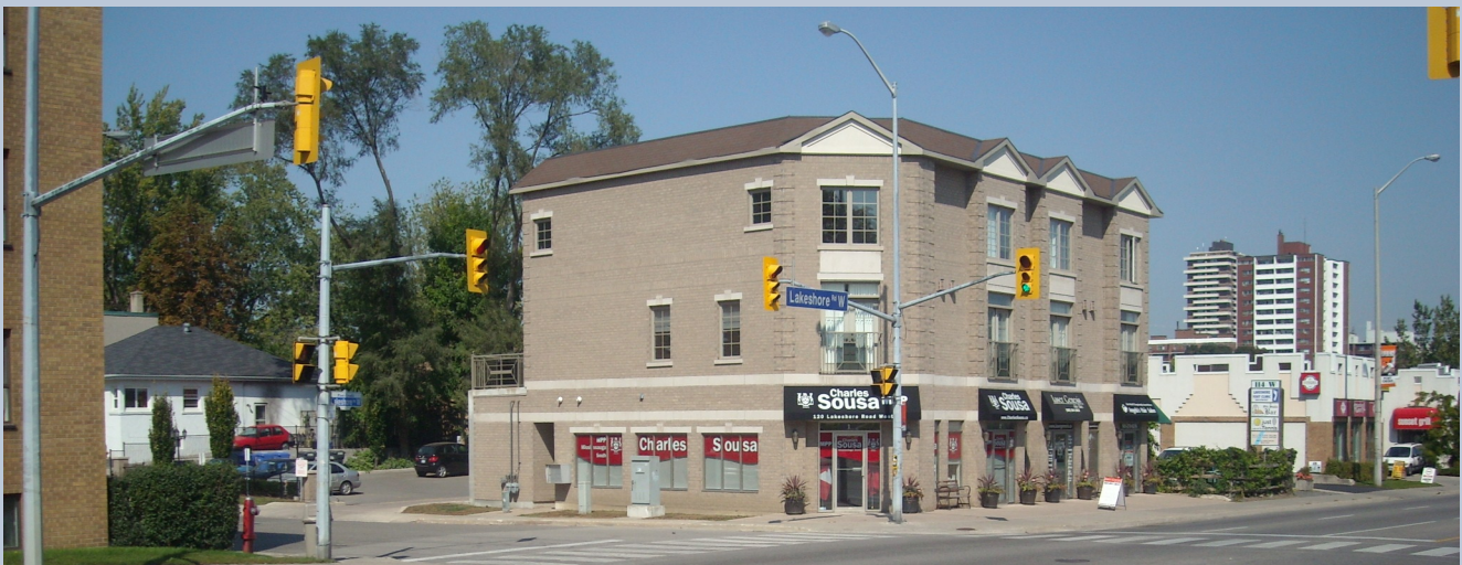
Figure B32 —Mainstreet Precinct, Mississauga Road and Lakeshore Road West. New construction.
