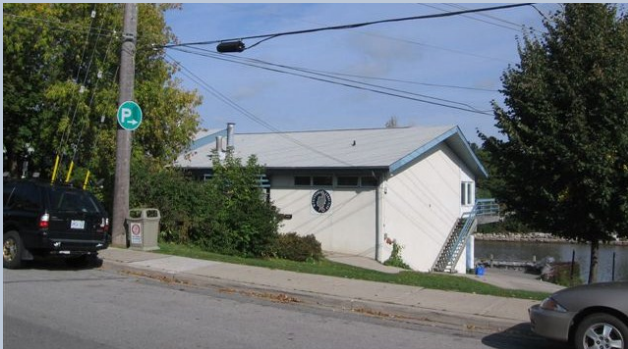
Figure B16 –Image of the Riverside Precinct
