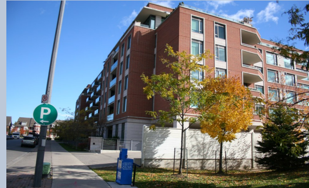
Figure B83 -Image of the Harbour Mixed Use Precinct
