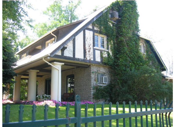
Figure B3 -Central Residential Precinct Image
