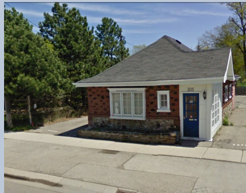
Figure C36 -305 Lakeshore Road West Designated
