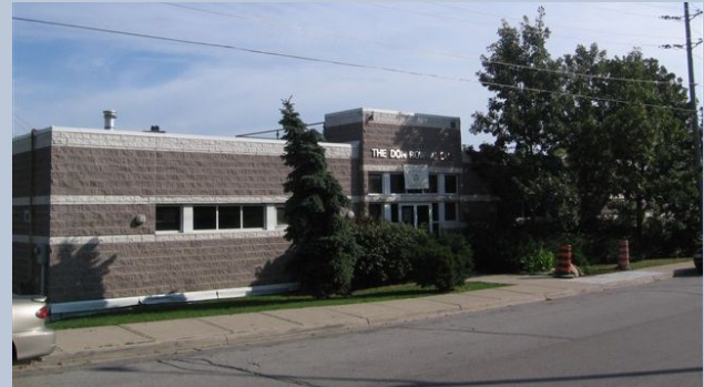
Figure B17 -Image of the Riverside Precinct
