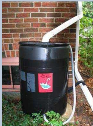
Figure D3 -Typical rain water barrel
