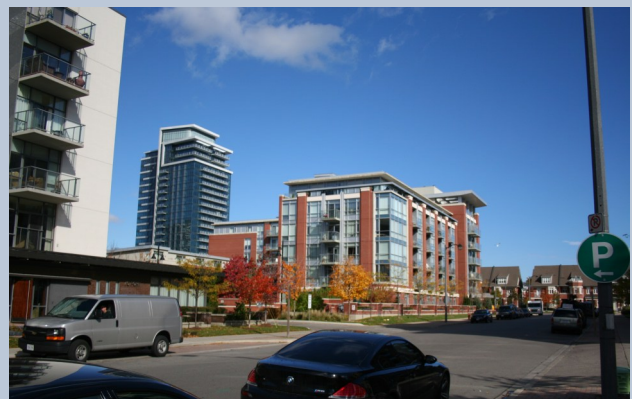
Figure B81 -Image of the Harbour Mixed Use Precinct
