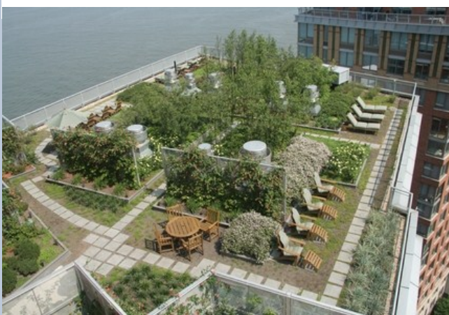
Figure B101 - Green Roof Example
