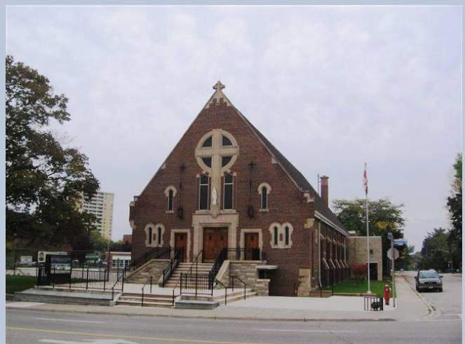
Figure B145- 141 Lakeshore Road West, Designated
