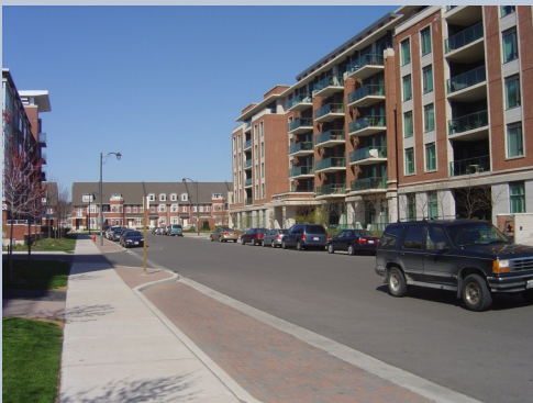
(top left) Figure B28 -Existing development south of Port Street East.
